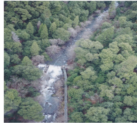
NORTH BATTLE CREEK FEEDER DIVERSION DAM
